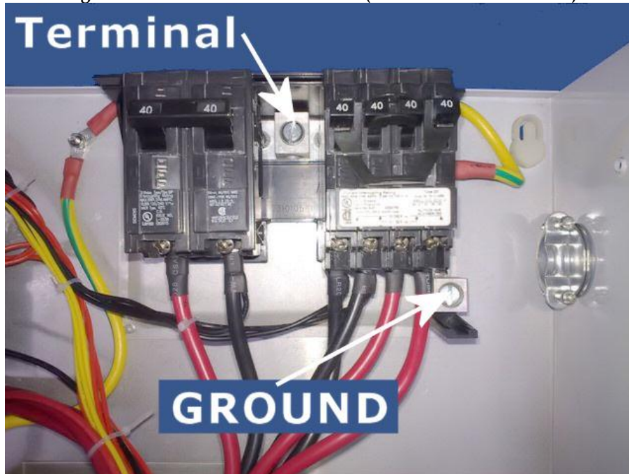
Figure 3 : Interior of the water heater (Models from 21 to 27 kW)
